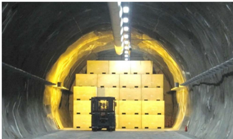
FIGURE 17: Disposal Vault at the Bataapáti Repository, Hungary [NOS 2014]
