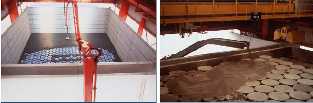
FIGURE 8: Backfilling of CSFMA LLW vault with concrete (L) and ILW vault with gravel (R) [NOS 2014]
