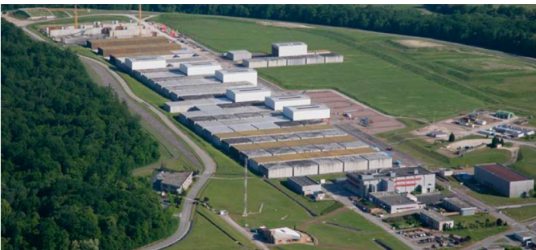
Aerial view of the Centre de l'Aube Repository for short-lived L&ILW, France
